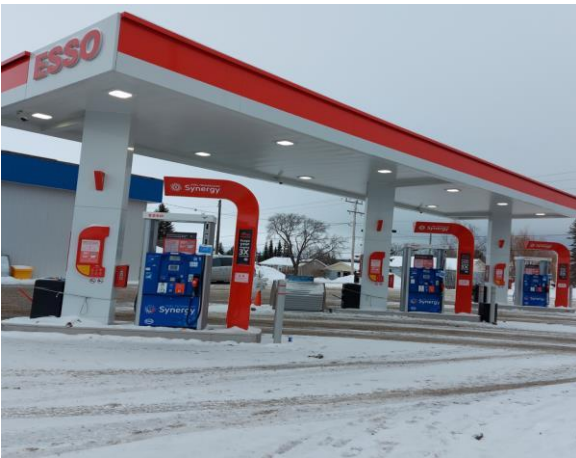
Gas Canopy Area
