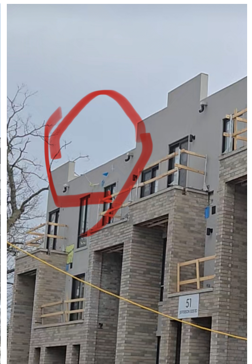
Photograph taken on April 29, 2025—16 months after the Receiver's appointment—clearly shows that no safety railing or warning signage was installed along the open roof edge, despite a drop exceeding 2.4 meters. This represents a serious breach of Ontario Regulation 213/91 (Construction Projects) and the Occupational Health and Safety Act (OHSA).
