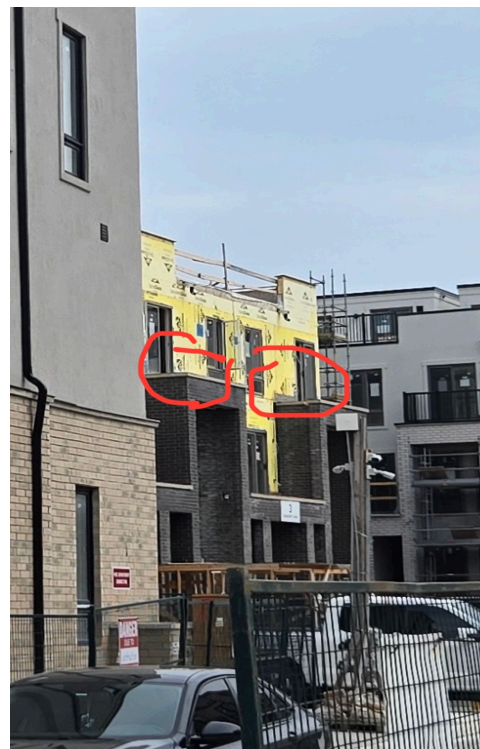
Photograph taken on April 29, 2025—16 months after the Receiver's appointment—clearly shows that no safety railing or warning signage was installed along the open roof edge, despite a drop exceeding 2.4 meters. This represents a serious breach of Ontario Regulation 213/91 (Construction Projects) and the Occupational Health and Safety Act (OHSA).
