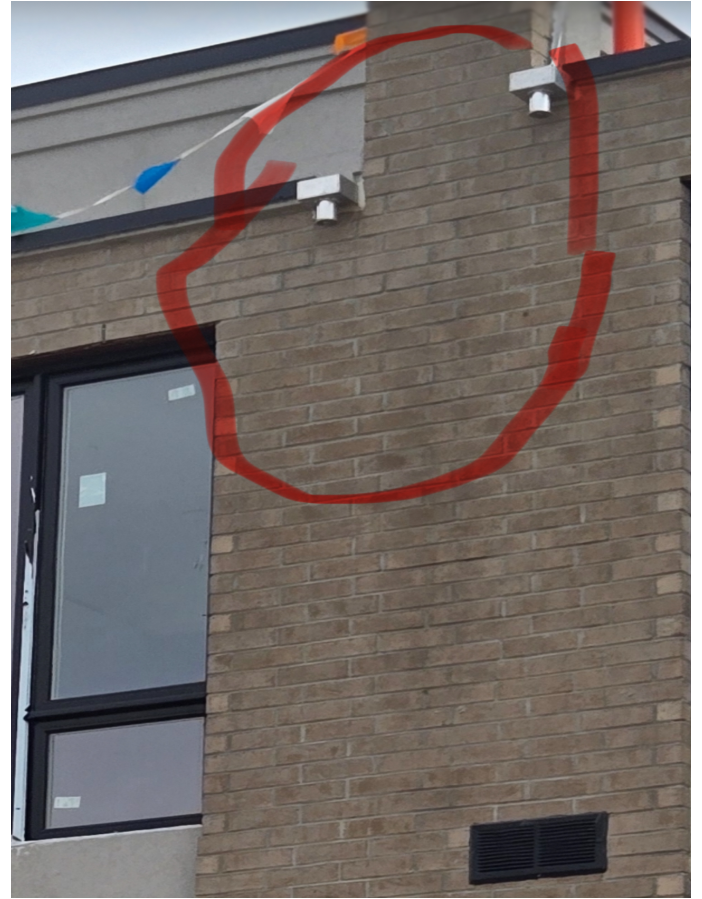
Photos taken on April 29, 2025 showing the water damage due to lack of drainpipe installation which should be installed a year before, the evidence of careless of the Reciever to preserve the asset value for the stakeholders.
