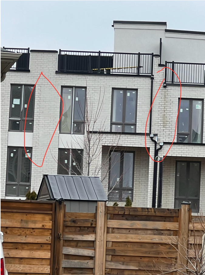
Photos taken on April 29, 2025 showing the water damage due to lack of drainpipe installation which should be installed a year before, the evidence of careless of the Reciever to preserve the asset value for the stakeholders.
