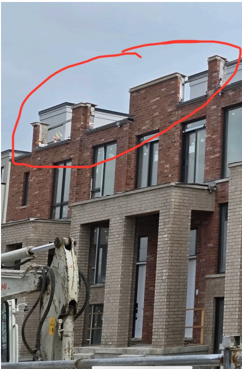
Photograph taken on April 29, 2025—16 months after the Receiver's appointment—clearly shows that no safety railing or warning signage was installed along the open roof edge, despite a drop exceeding 2.4 meters. This represents a serious breach of Ontario Regulation 213/91 (Construction Projects) and the Occupational Health and Safety Act (OHSA).
