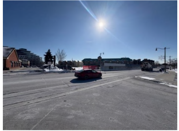
View of subject property looking southwest along Lakeshore Road West
